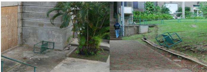
Racks out of place
